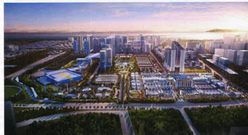
Aerial view of the 247-acre Aspen Vision City in Batu Kawan
